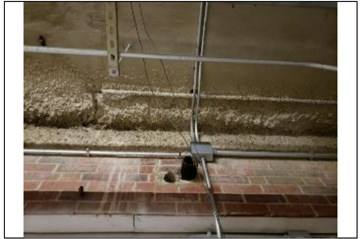
10. Spray-on fireproofing present, previously tested and had no asbestos detected.
