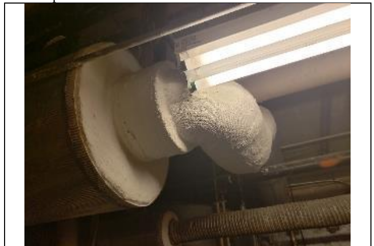
6. White canvas insulation on exhaust pipe in Room 125, no asbestos detected.
