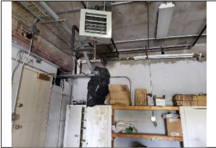
9. Basement Room B16C.
